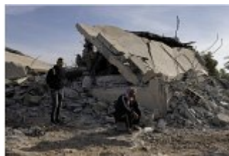
Villagers stand next to the rubble of destroyed buildings in Umm Al-Hiran, Nov. 14, 2024. (Oren Ziv)
